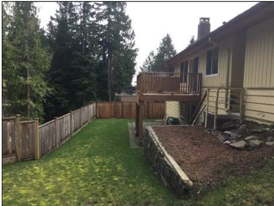
Photograph 5. 1582 Merlynn Crescent – Looking south at backyard. Wood fence is located on top of the retaining wall at the escarpment crest.
