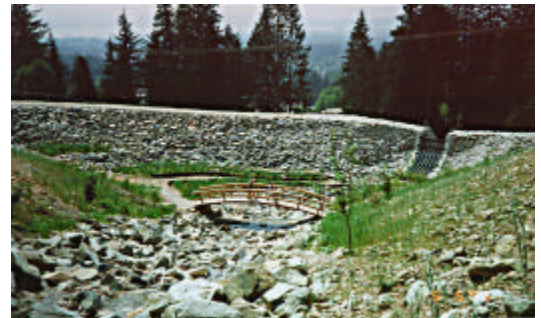
Upper Mackay Creek Debris Basin
