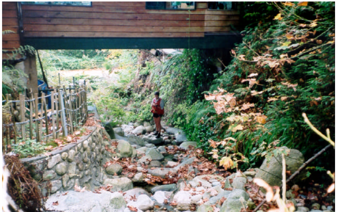
Photo P-4 House addition constructed across Panorama Creek above Panorama Drive. October 2001.
