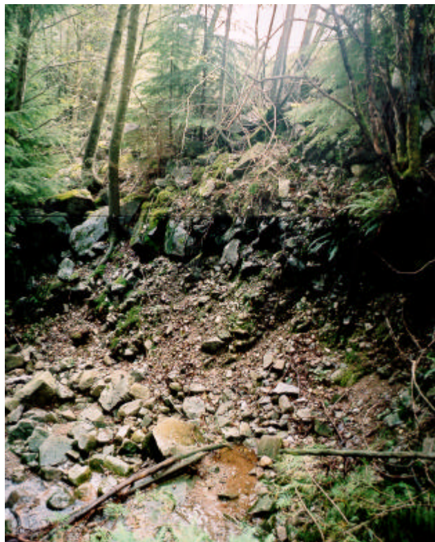
Photo F-2 Bank erosion of fill slope at the first switchback of Mount Seymour Road. Approximate elevation 390 m. October 2001.
