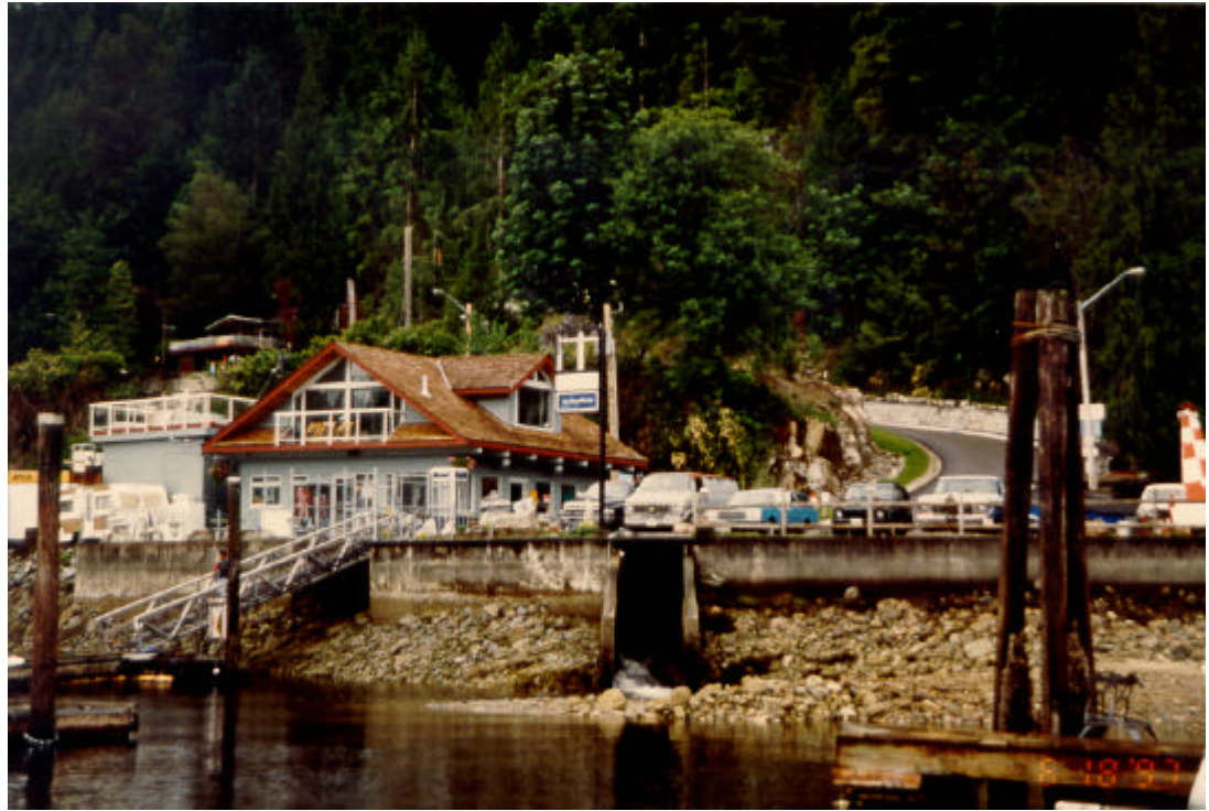
Photo F-11 Deep Cove Marina and the box culvert outlet for Francis Creek. June 1997.
